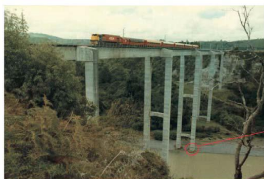
Figure 2: Application of rocking motion and energy dissipation devices at the base of the southern Rangitikei railway bridge (Cornak, 1998)
